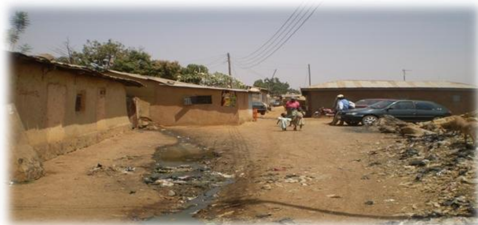
Fig. 1: Sewage disposal from houses into the streets Source: Authors Fieldwork, 2012
